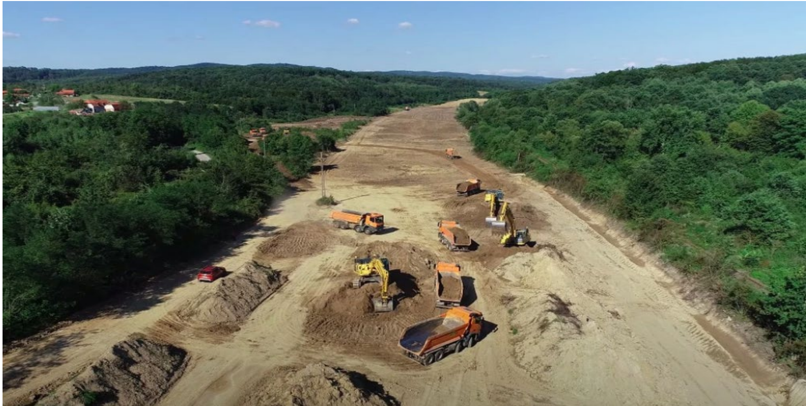
Highway construction nearby
